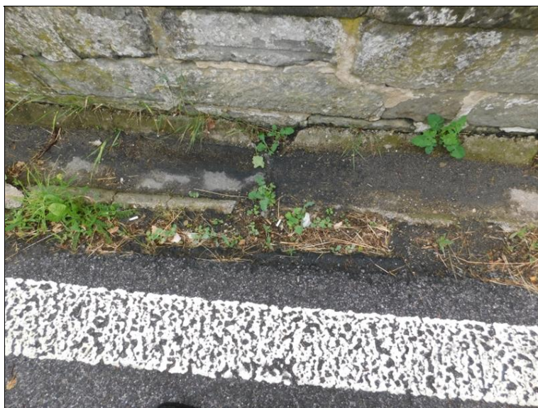
Deformace krajnice, uchycená vegetace.
